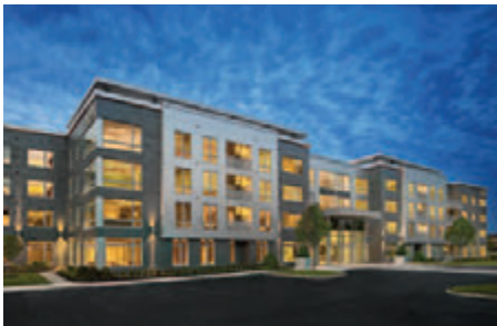
90 Park Avenue Florham Park
