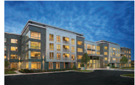
90 Park Avenue Florham Park
