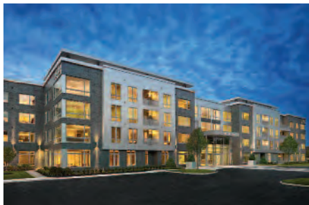
90 Park Avenue Florham Park
