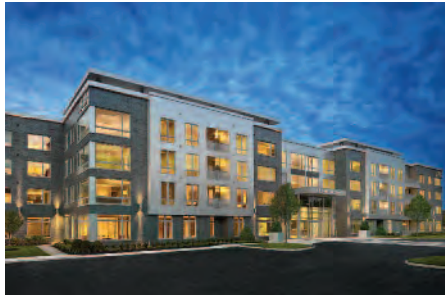
90 Park Avenue Florham Park
