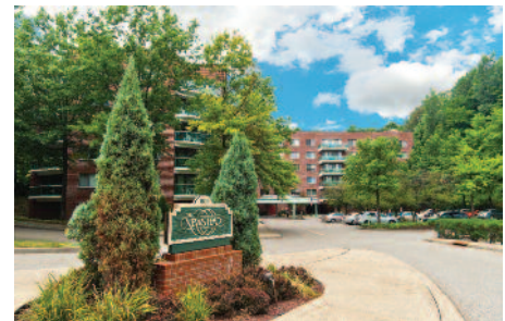
609 S. Orange Ave., 2M South Orange $325,000
